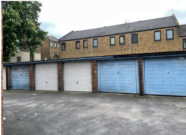
Figure 6 – Single storey garages as Existing
