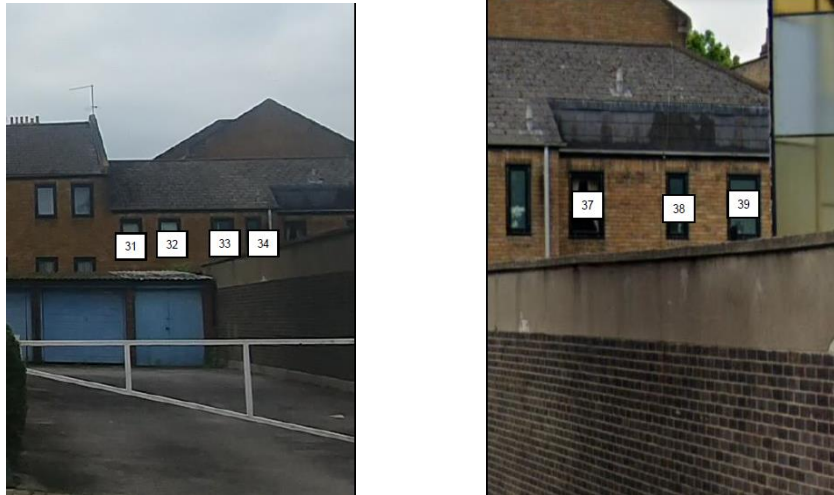
Figure 14 – Windows tested at 10-17 Searle Place
