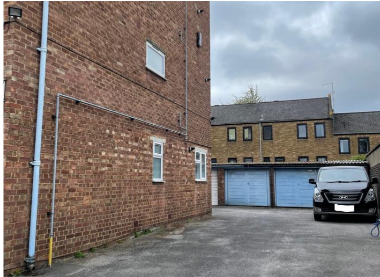
Figure 5 – Existing accessway leading to Garages at the rear
